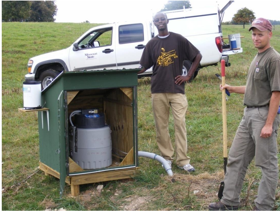
Photo 11. Auto-sampler and Rain Gage Installation (October 2008)
