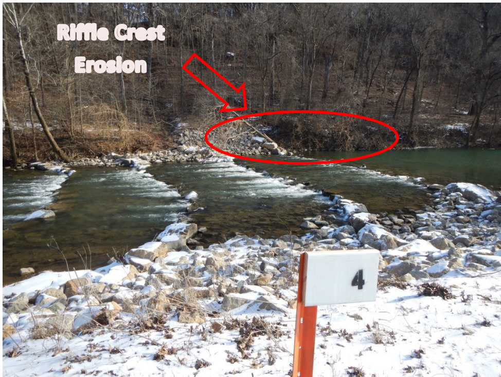
Photo 10. Erosion along the right bank near riffle structure crest (1/21/16).
