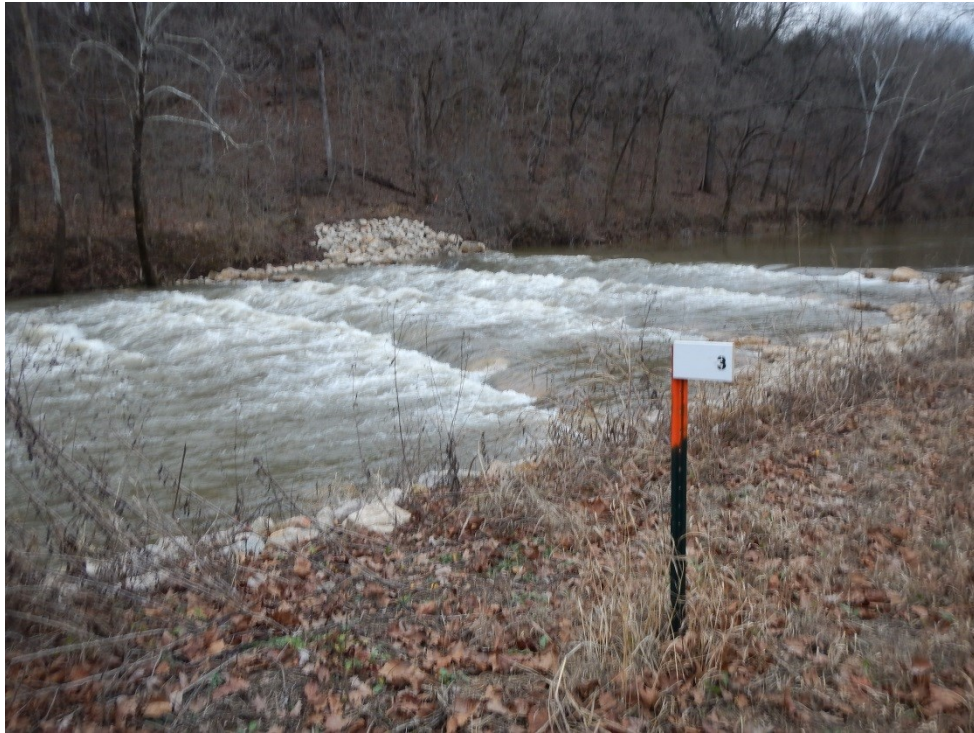
Photo 1. Constructed riffle at Transect 3 (12/14/15).
