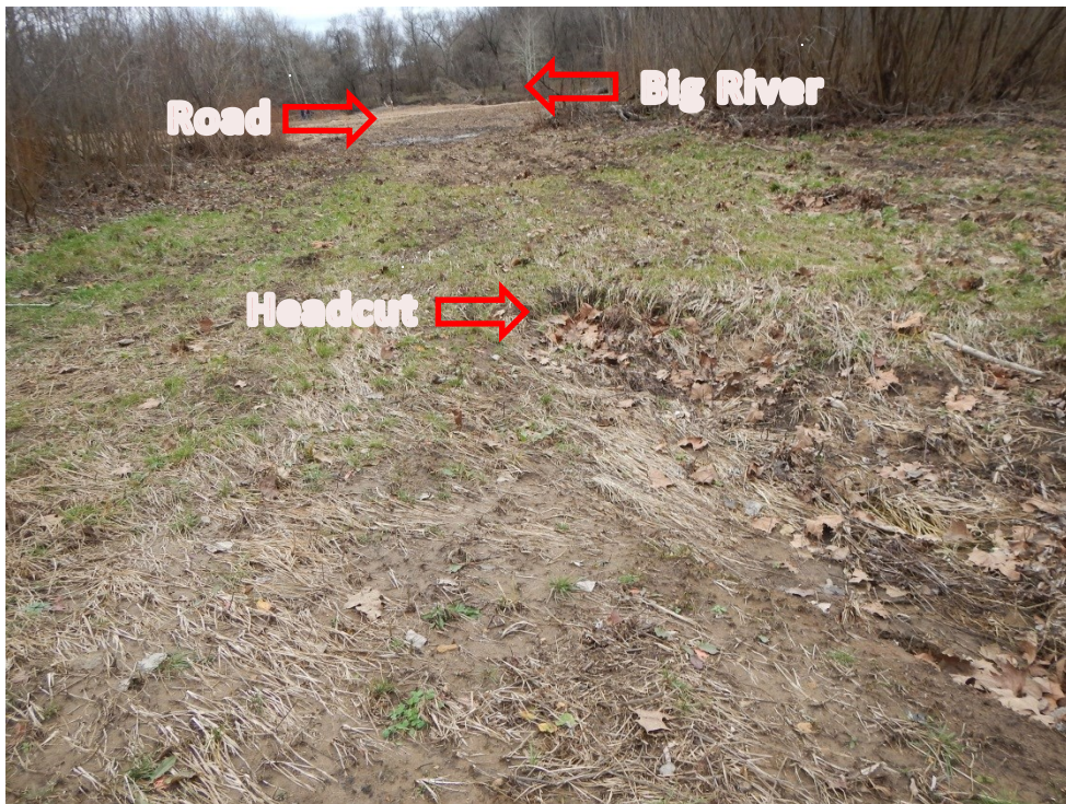
Photo 4. Basin channel opening from the upper basin with headcut (12/14/15).
