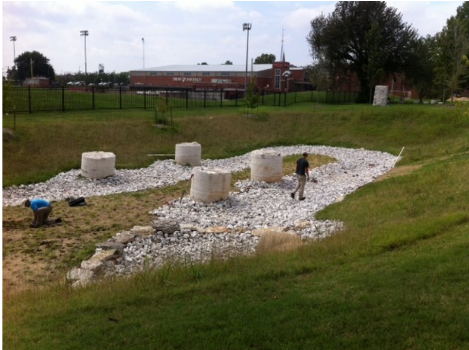
Photo 8. Drury basin post-retrofit
