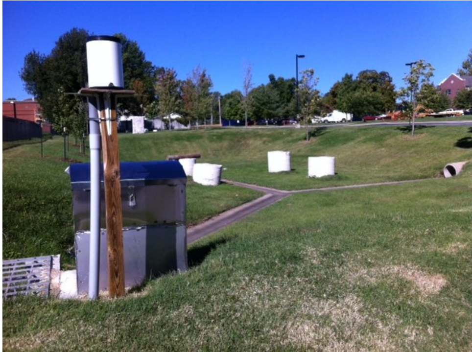
Photo 7. Drury basin pre-retrofit
