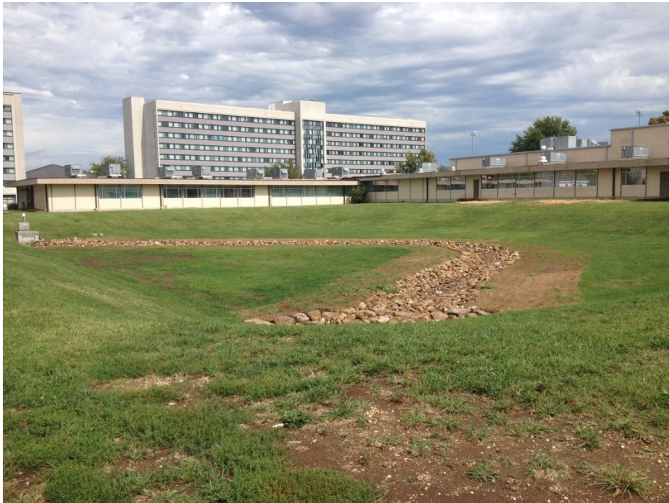
Photo 12. Greenwood basin post-retrofit
