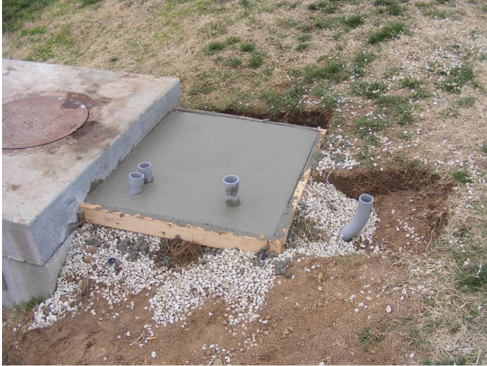
Photo 3. Concrete pad after the pour with trench to rain gage
