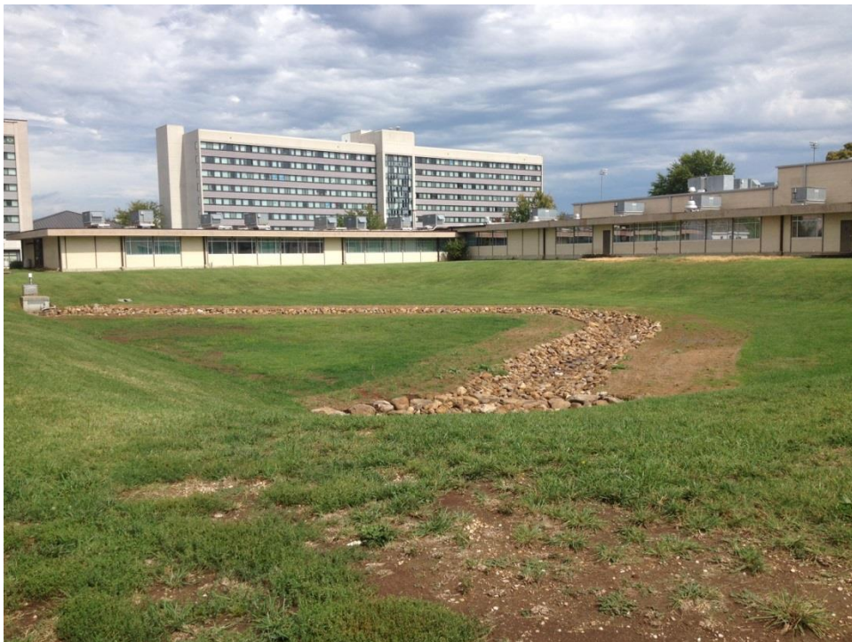
Photo 10. Greenwood basin post-retrofit
