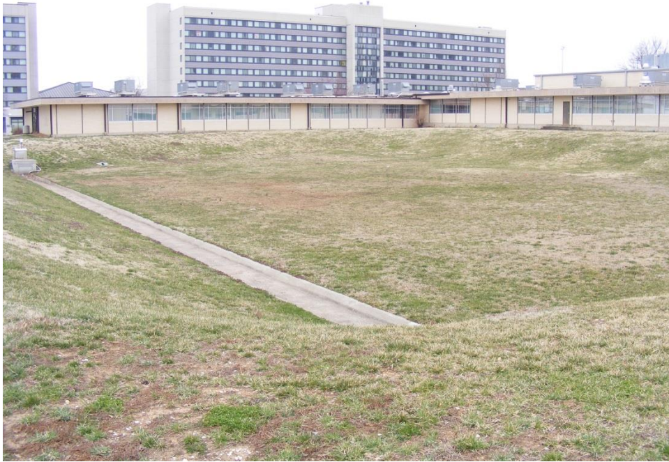
Photo 9. Greenwood basin pre-retrofit
