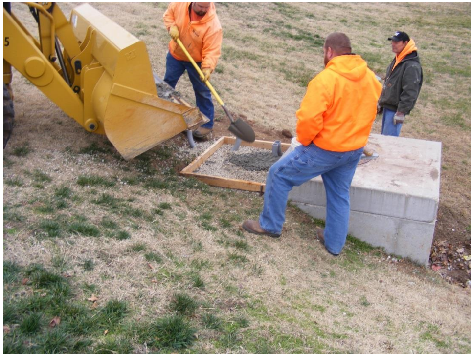
Photo 2. Pipe rough in, concrete forms and pad pouring by City of Springfield crews
