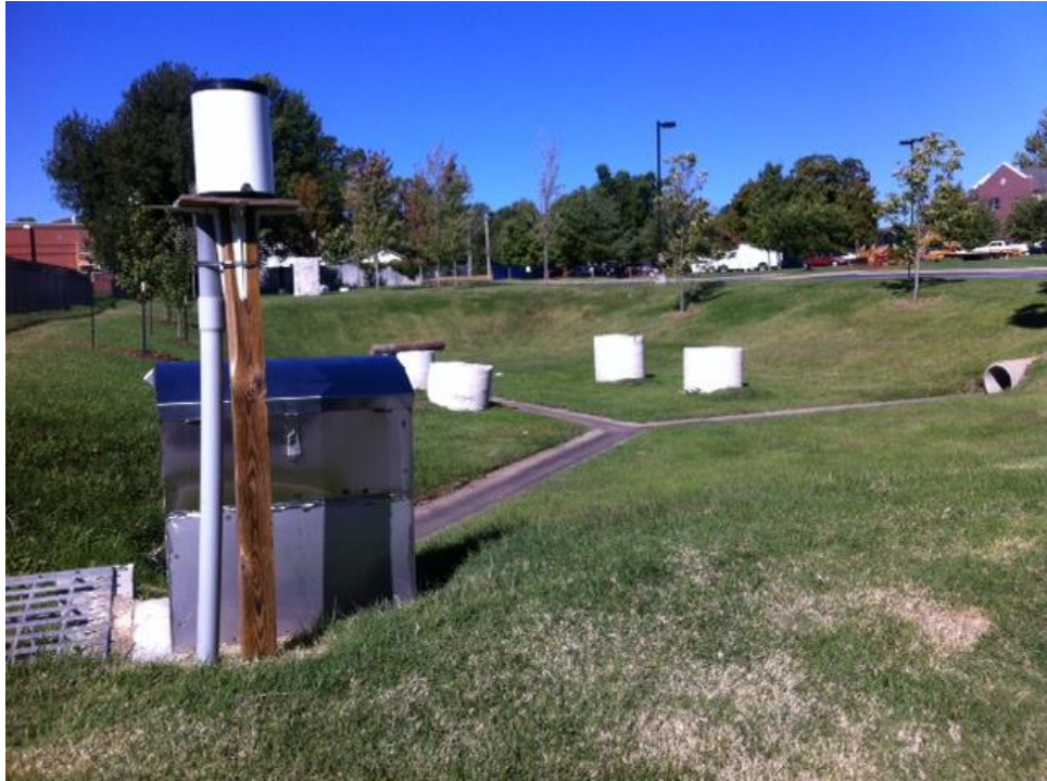
Photo 7. Drury basin pre-retrofit
