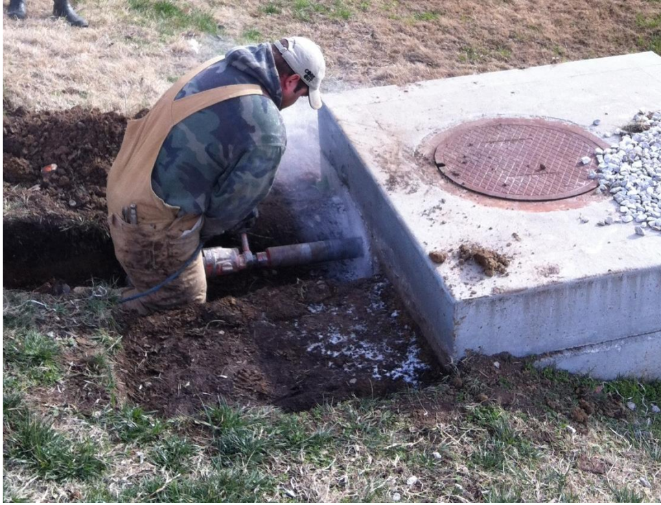
Photo 1. Excavation and concrete cutting for installation of the monitoring station
