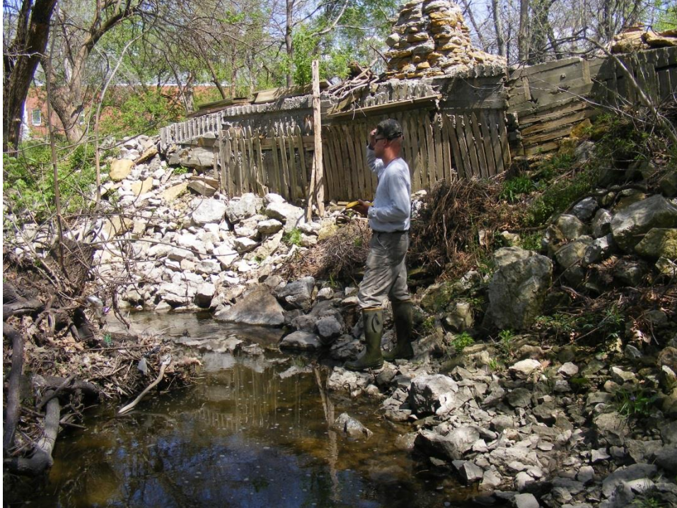
Photo 14. Local residents are trying to protect their land in areas where bank erosion threatens their property.
