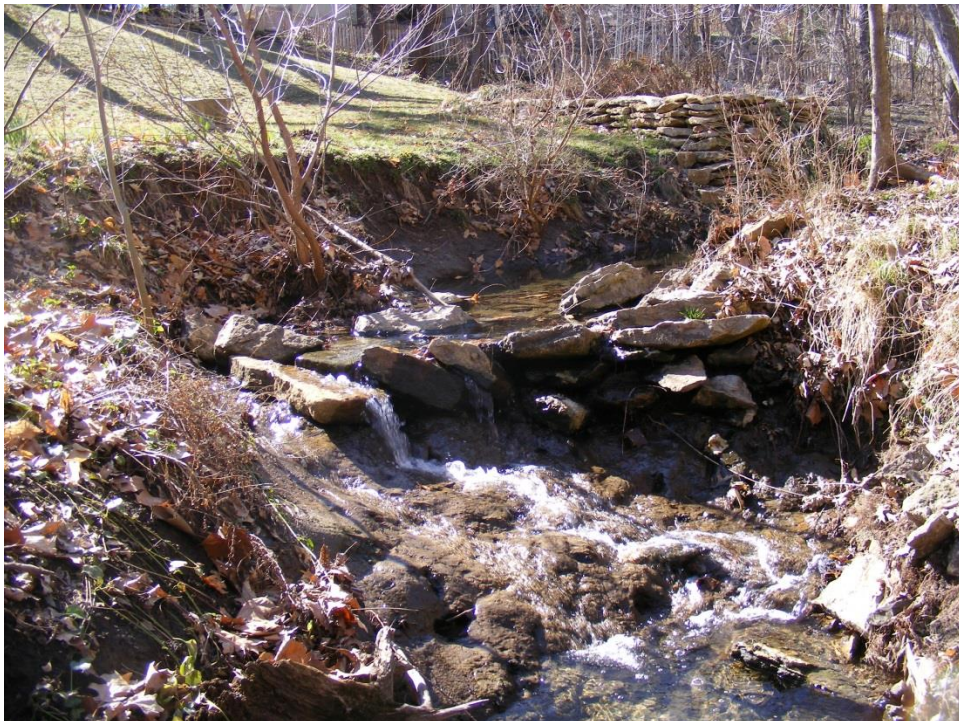
Photo 12. Headcuts are progressing upstream in most of the tributaries.
