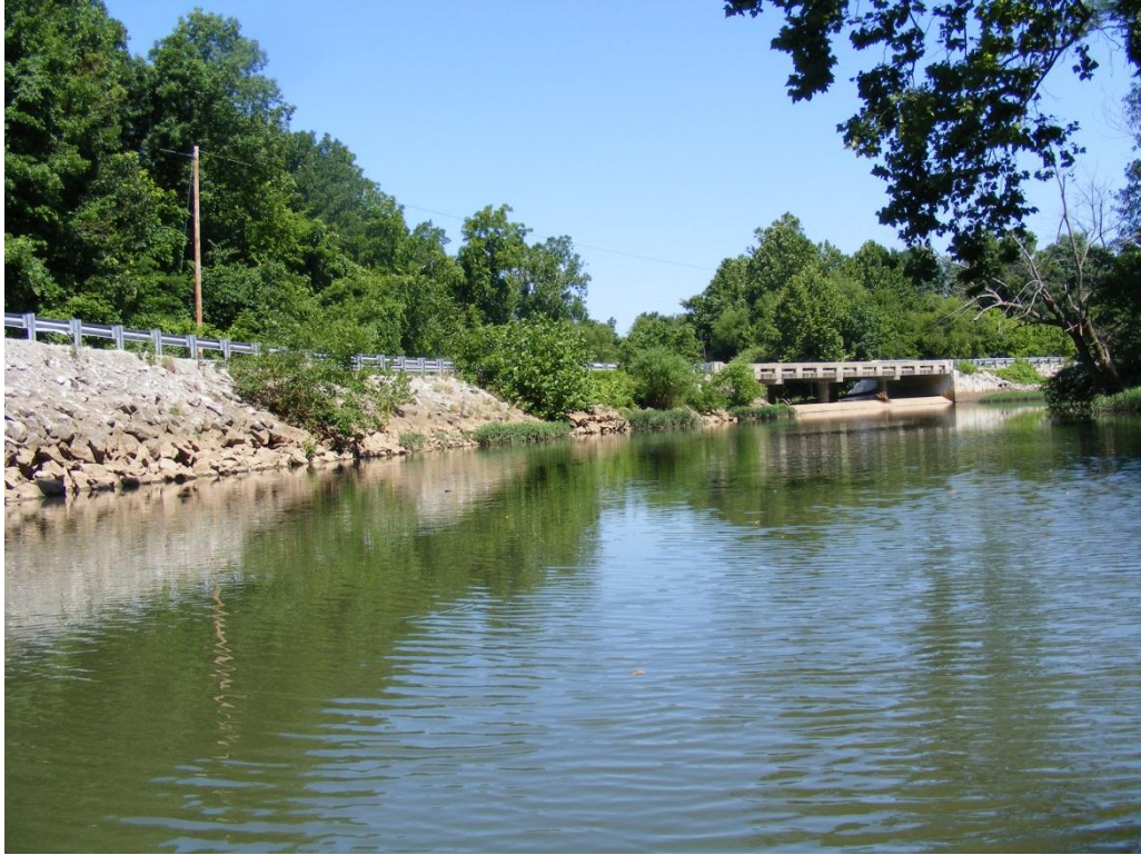
Photo 3. Rip rap along Cox Road at station 2.3 km.
