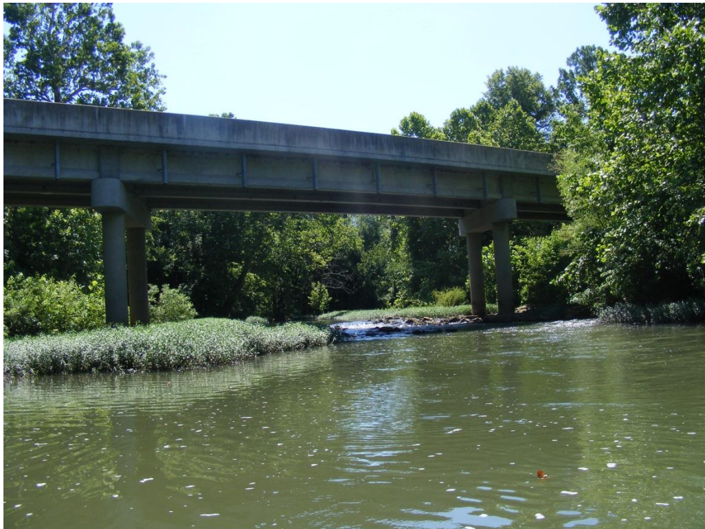
Photo 4. Cox Road Bridge at station 2.7 km
