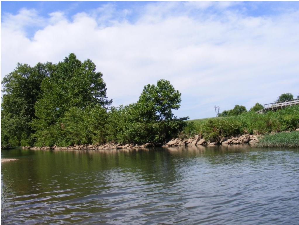
Photo 9. Rip rap lined bank adjacent to the golf course near disturbance reach at station 4.6 km
