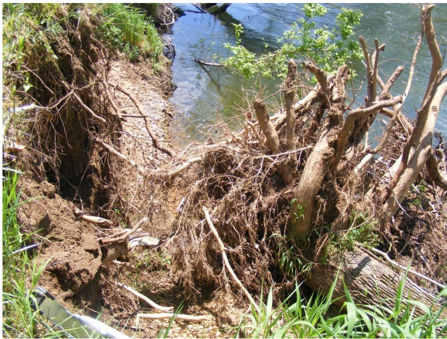
Photo 10. Recently downed tree after bank failure, May 2013.
