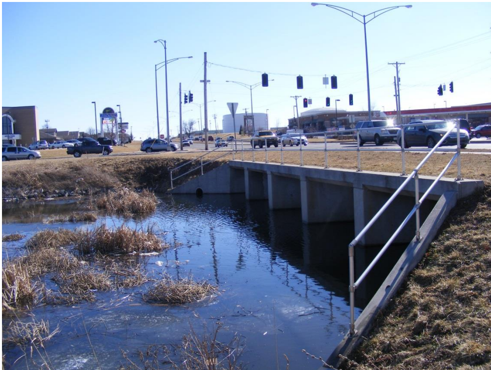
Photo 2. KAN monitoring site looking south along Kansas Expressway.
