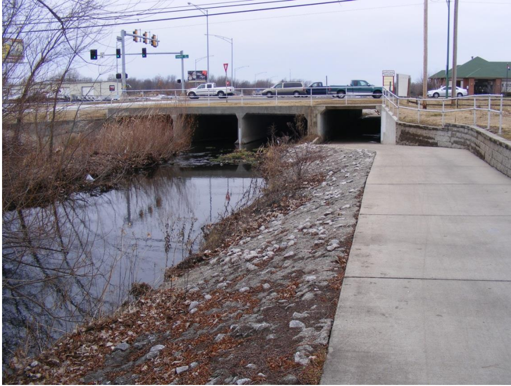
Photo 1. CAM monitoring site looking west toward Campbell Avenue.
