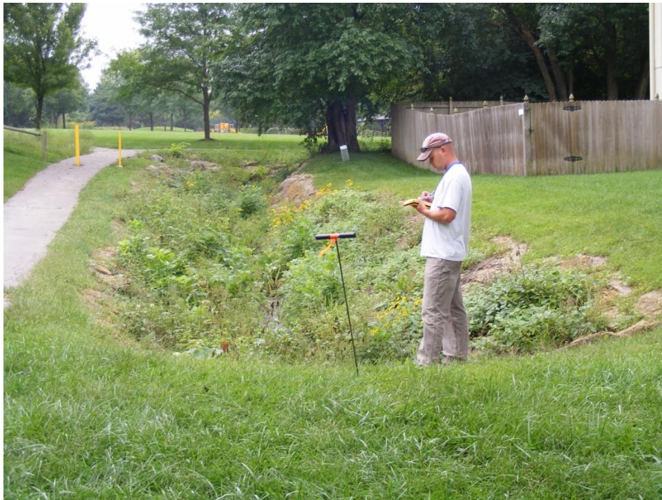
Photo 4. R3 - Rip-rap and culvert inlet St. 7,030 looking upstream (Sept. 2009)
