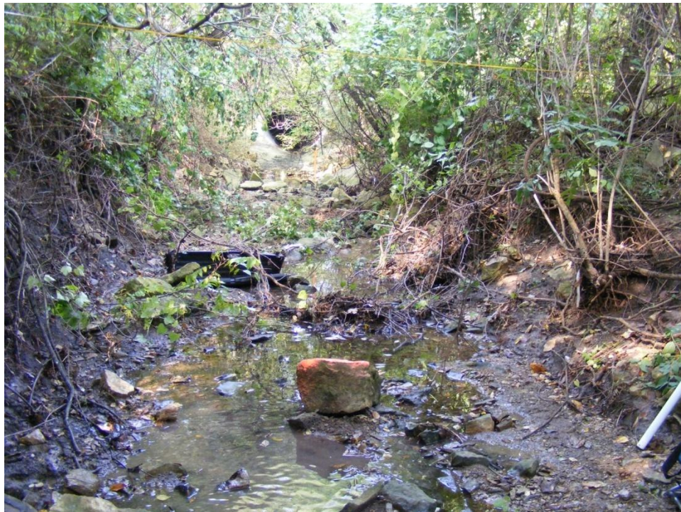
Photo 24. R11 – xs 11, St. 3,710 ft looking upstream (Sept. 2009)
