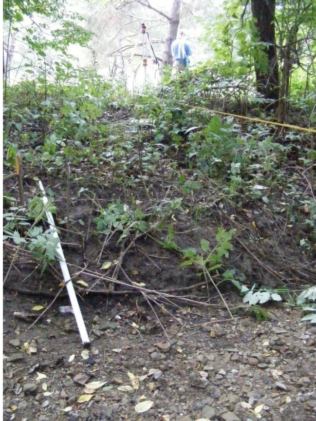
Photo 23. R9 – xs 10 St. 4,260 ft left bank (Sept. 2009)
