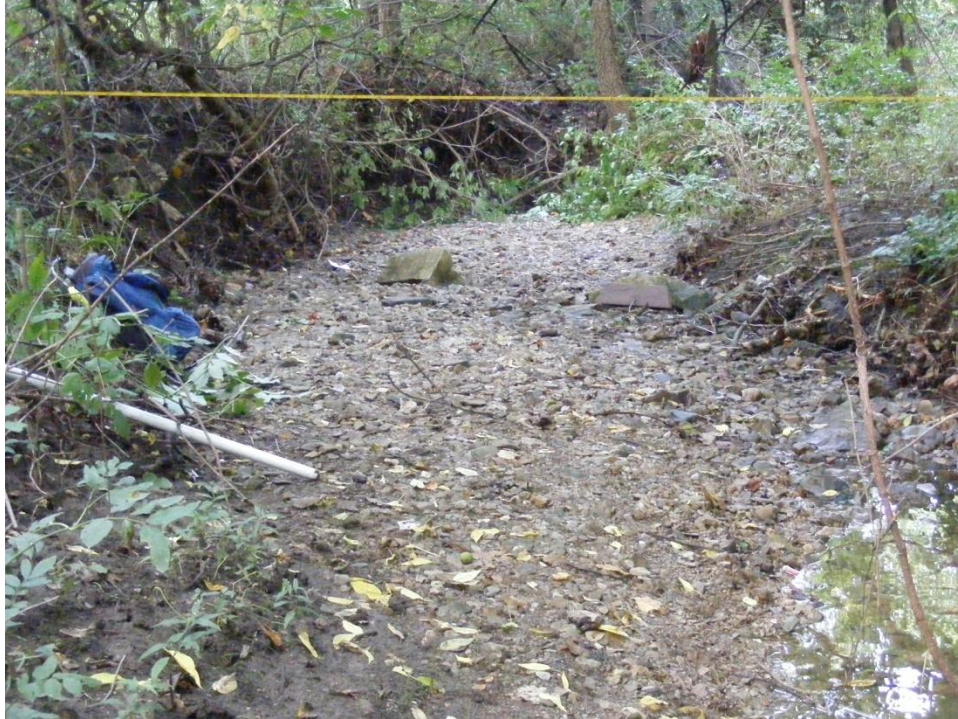
Photo 21. R9 – xs 10, St. 4,260 ft looking upstream (Sept. 2009)
