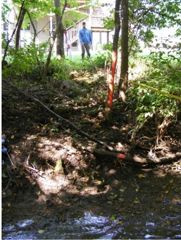
Photo 39. R14 – xs 14 St. 2,140 ft left bank (Sept. 2009)
