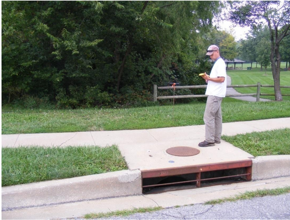
Photo 1. R1-A Start of Project St. 7,870 ft looking downstream (Sept. 2009)
