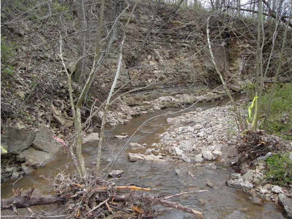
Picture 9. Looking downstream at distance 2500
