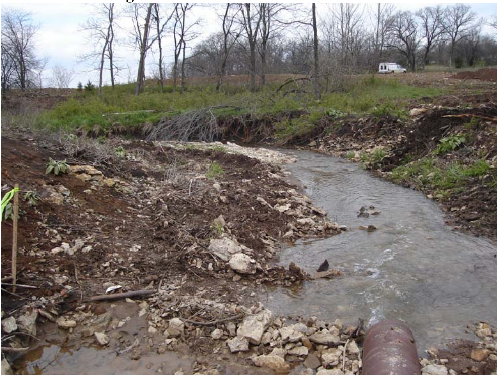
Picture 6. Looking downstream at distance 2800
