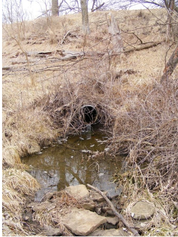
Photo 1. Pond dam outlet begins SR-1 (Feb. 2008)
