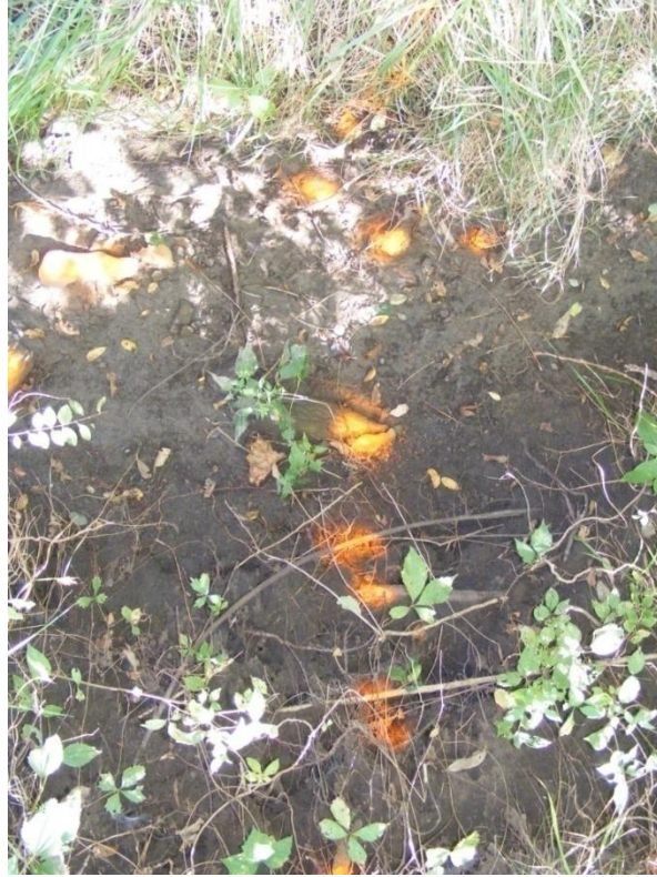
Photo 37. PA-8 installation Sept. 2007
