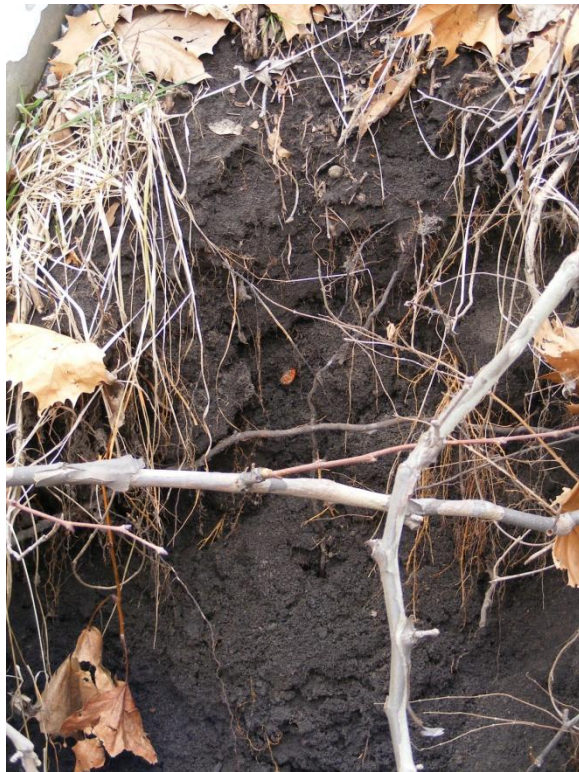
Photo 26. PA-2 as of Feb. 2008 showing upper bank slump.
