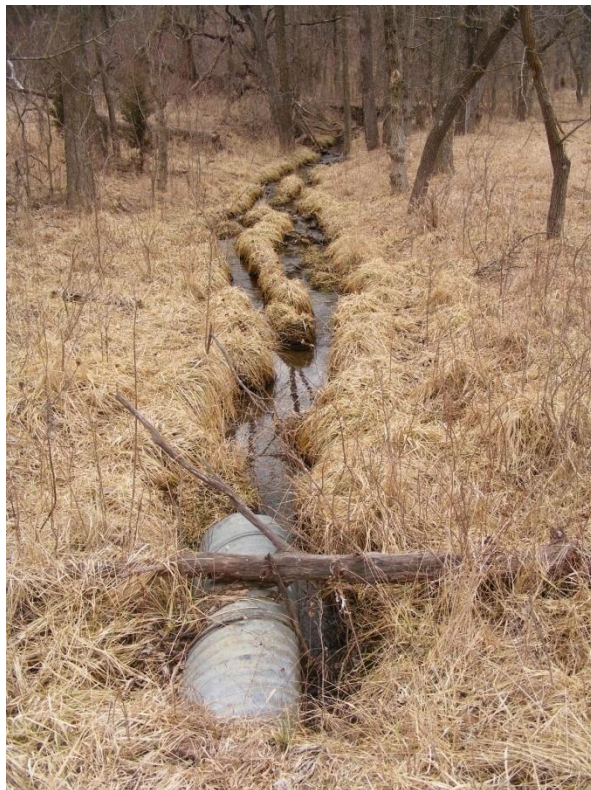
Photo 20. SR-11b looking downstream from culvert (Feb. 2008)
