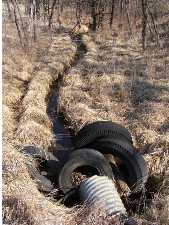
Photo 19. SR-11a looking upstream from culvert (Feb. 2008)
