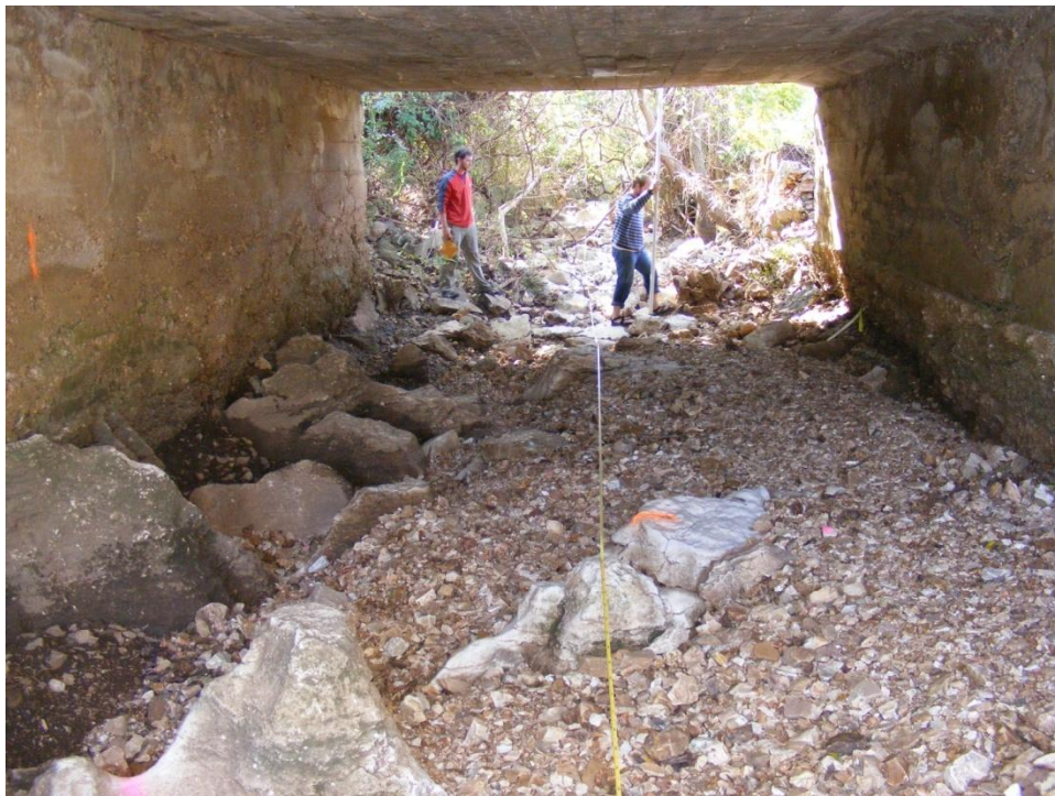
Photo 6. Looking downstream at SR-2 near station 900 feet (10/16/2008)
