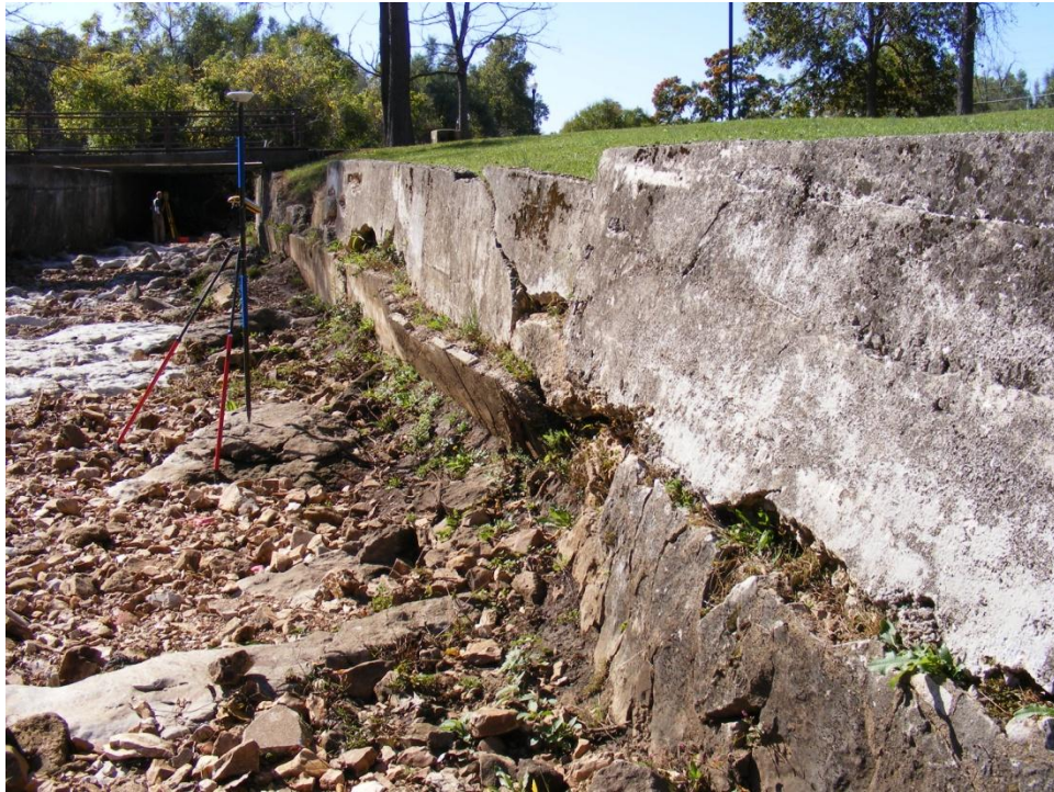
Photo 4. Looking downstream at SR-3 near station 1,050 feet (10/16/2008)
