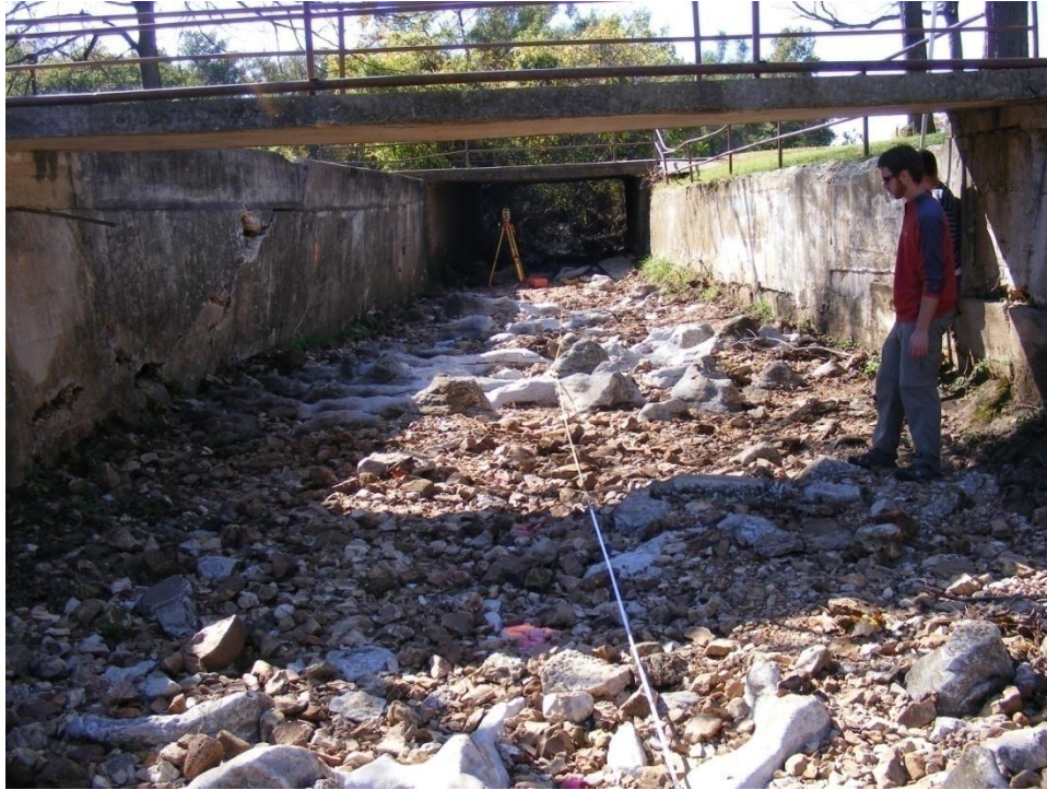
Photo 5. Looking downstream at SR-2 near station 1,000 feet (10/16/2008)
