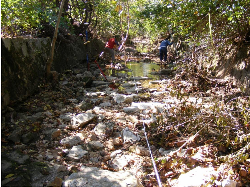
Photo 11. Looking downstream at SR-1 near station 470 feet (10/16/2008)
