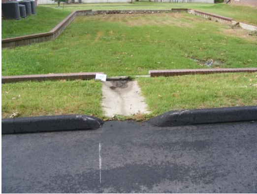
Parking lot and outfall above sample 37
