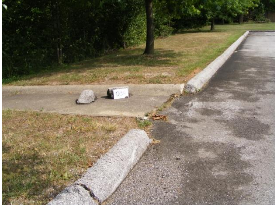
Parking lot and outfall above sample 34
