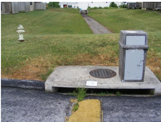
Parking lot and outfall above sample 36
