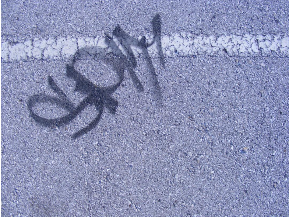
Asphalt Lot (Unsealed)
