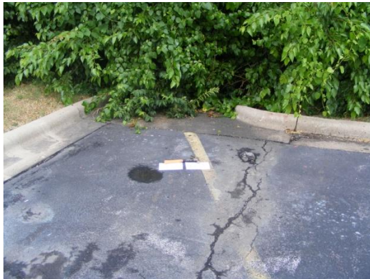
Parking Lot near outfall above samples 32 and 33
