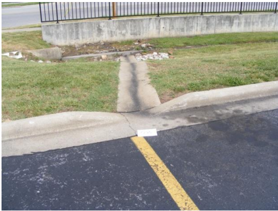
Parking lot and outfall above sample 35
