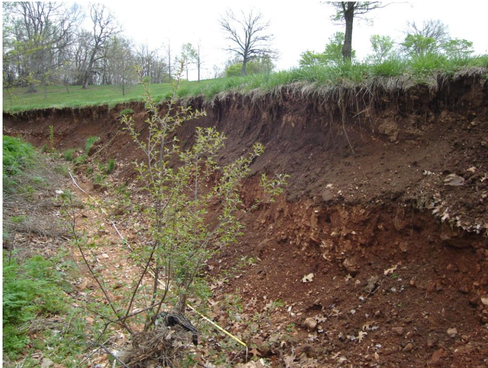
Picture 6 – Eroding bank along long bend at 500ft (sub-reach #3)
