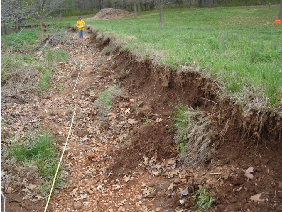
Picture 11 – Lower channel banks at 300ft (sub-reach #4)
