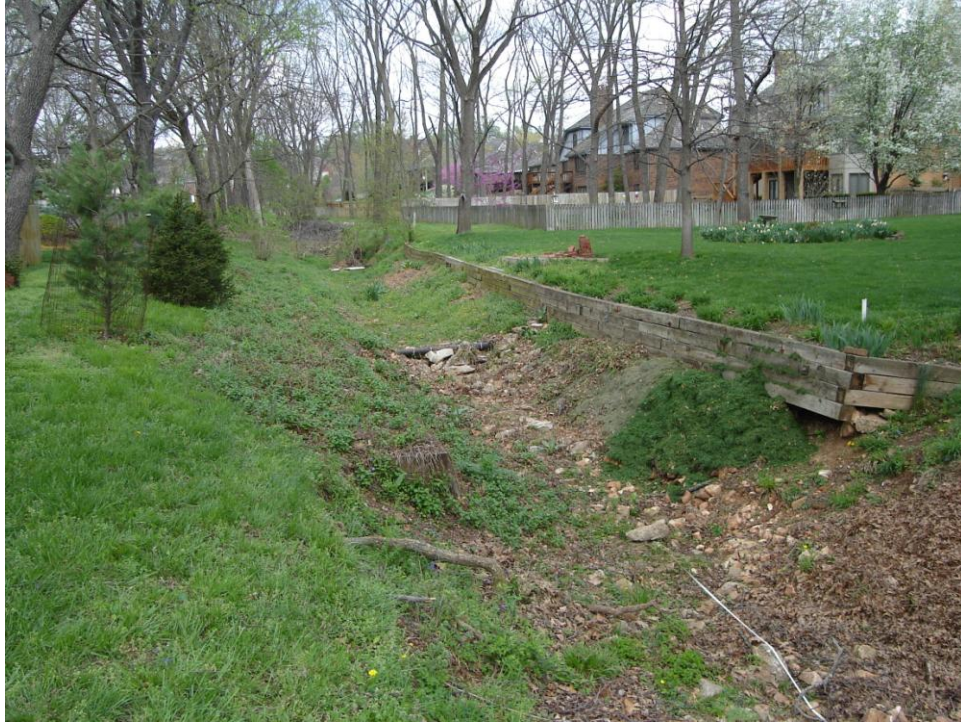
Picture 1 – Looking upstream at 800ft (sub-reach #1)
