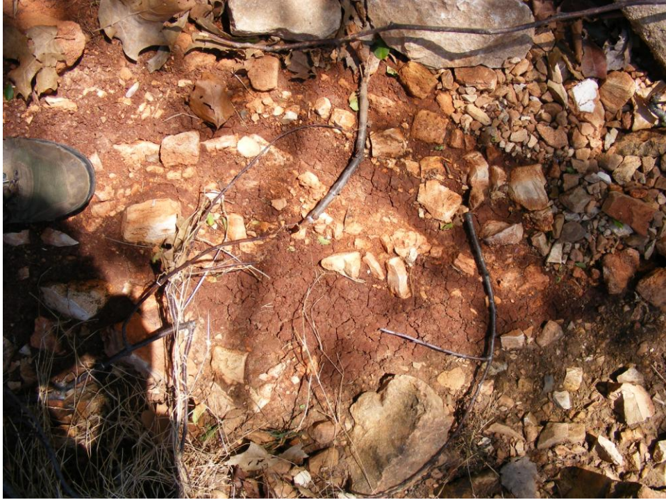
Picture 31 - Scoured residuum in plunge pool (4-29-08)
