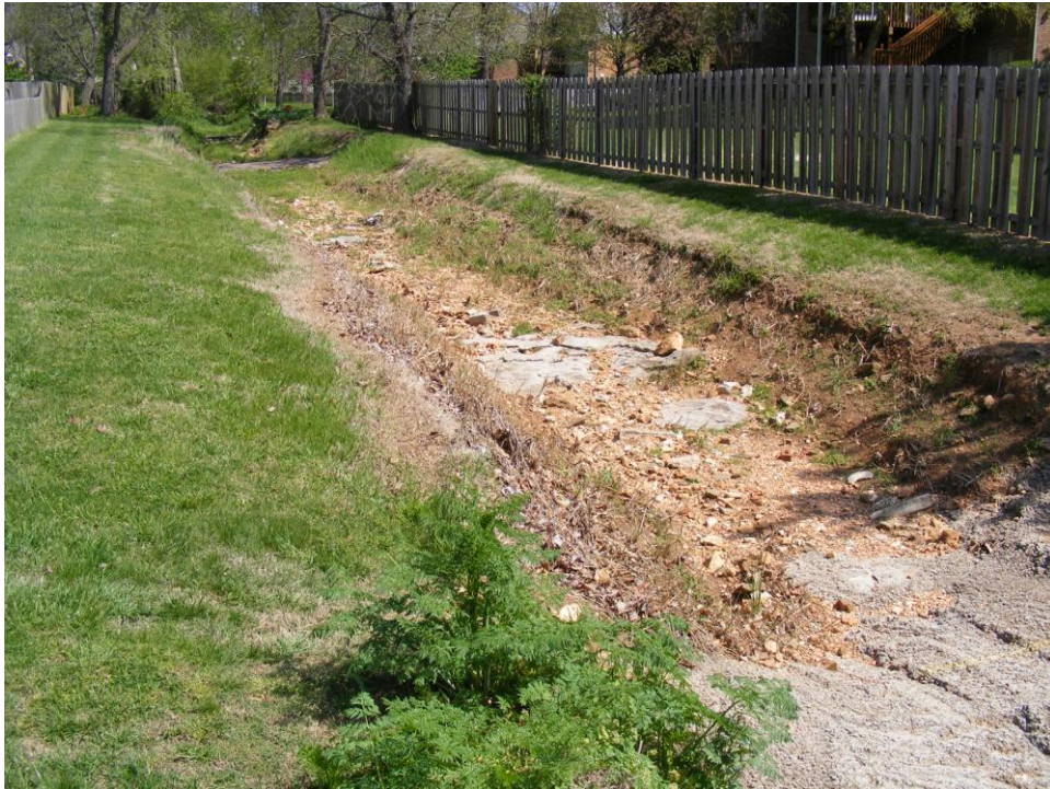
Picture 26 - Grass channel (SR #1) (4-29-08)
