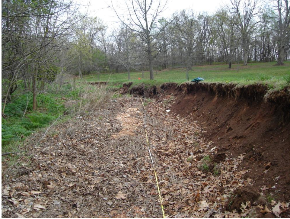
Picture 7 – Point bar on left (under leaves) at 450ft (lower end of sub-reach #3)
