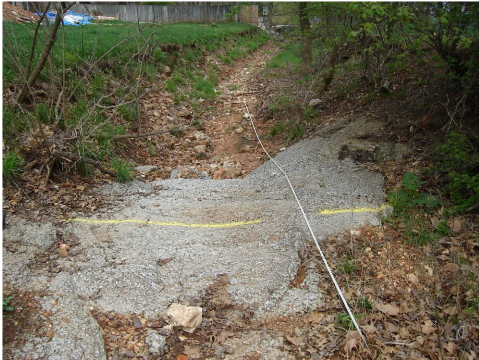
Picture 14 – Concrete bed obstruction marking end of study reach at 0ft
