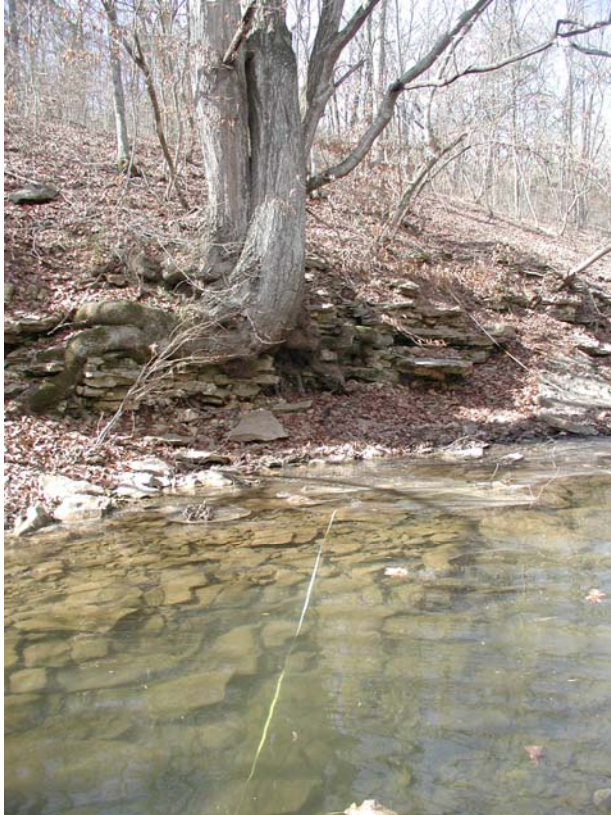
Picture 26. Bedrock bluff and colluvium along south bank (860 m)
