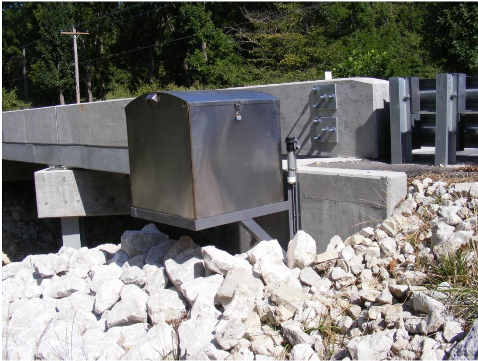
Photo 2. Sampler box installed on the east downstream wing wall at Site 1.
