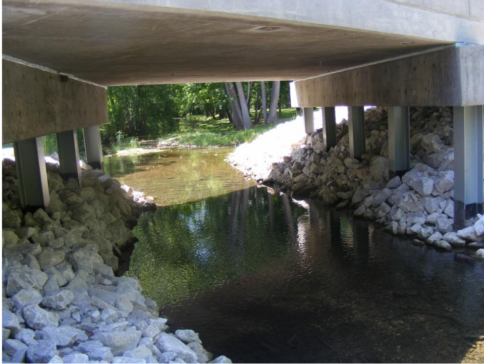
Photo 1. Site 1 at State Highway YY Bridge looking downstream.
