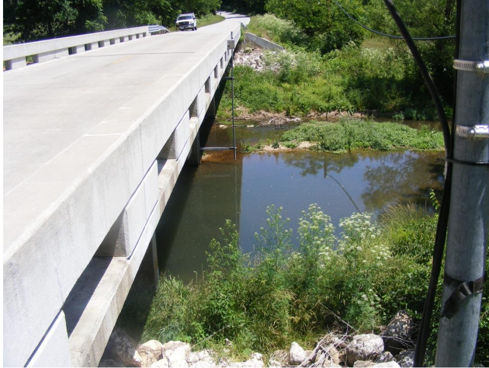
Photo 5. Site 3 at the Farm Road 148 Bridge looking east.
