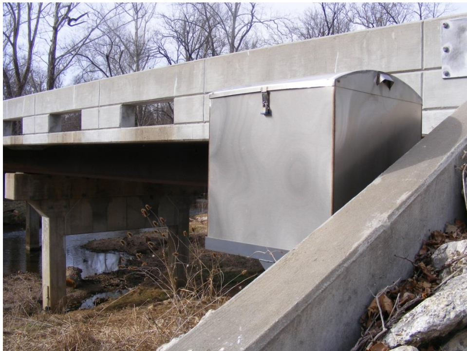
Photo 6. Sampler box installed on the downstream east wing wall at FR 148.
