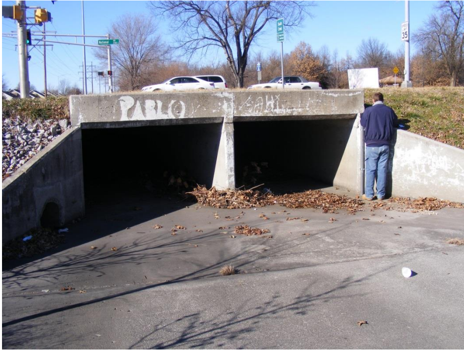
Photo 1. Site NAT upstream of National Avenue.
