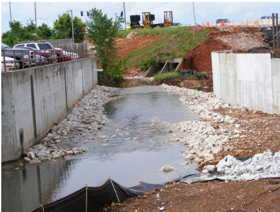
Photo 52. SR-14 upstream of National in the construction reach (station 3,700 ft).
