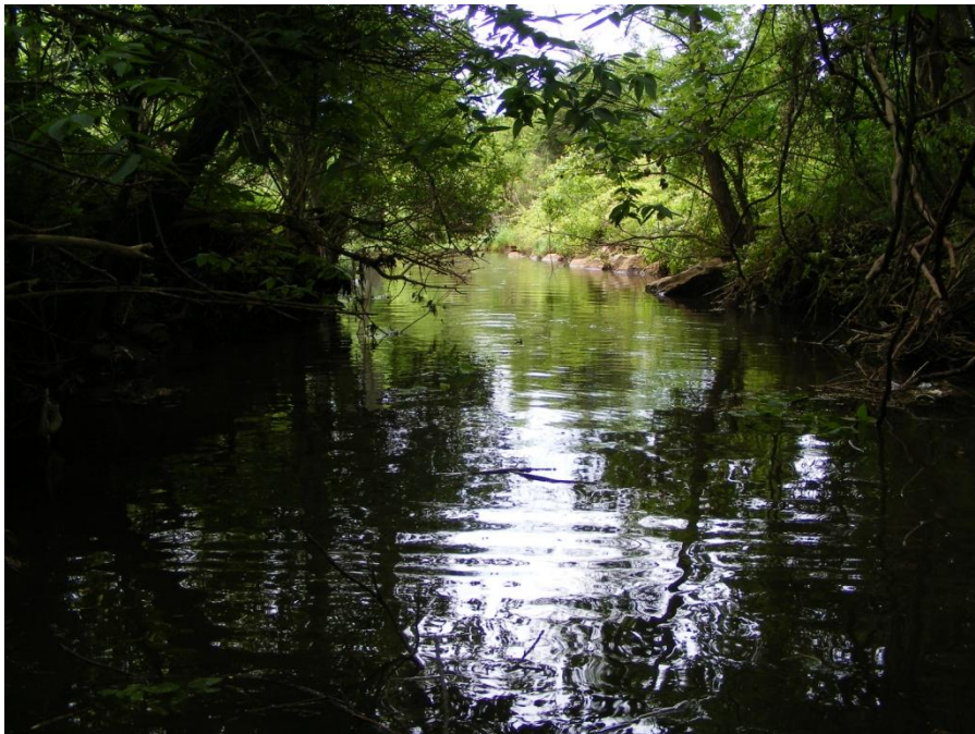
Photo 6. SR-2 pooled area upstream of concrete liner at cross-section #2 (station 225 ft) looking downstream.
