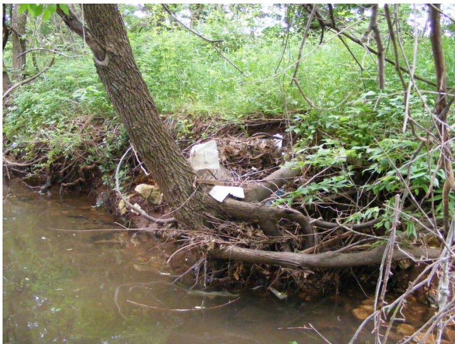
Photo 8. SR-2 cross-section #2 (station 225 ft) left bank.
