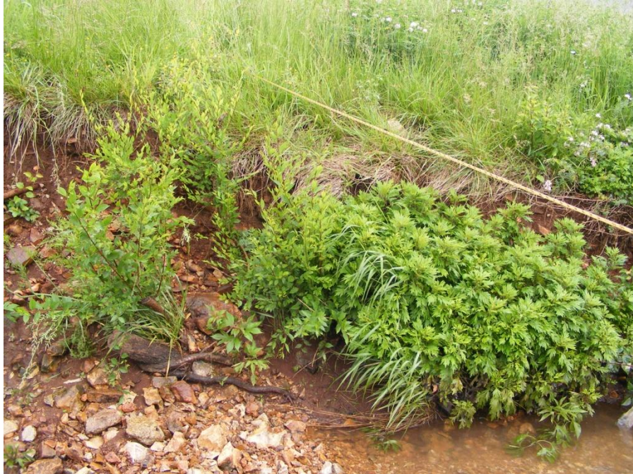
Photo 31. SR-8 cross-section #5 (station 1,340 ft) right bank.
