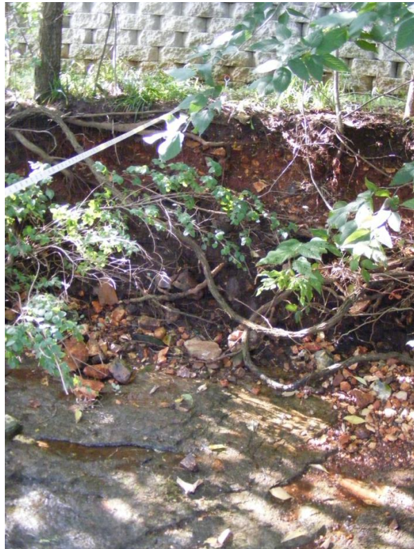
Photo 26. SR-5 cross-section #4b (station 825 ft) right bank.
