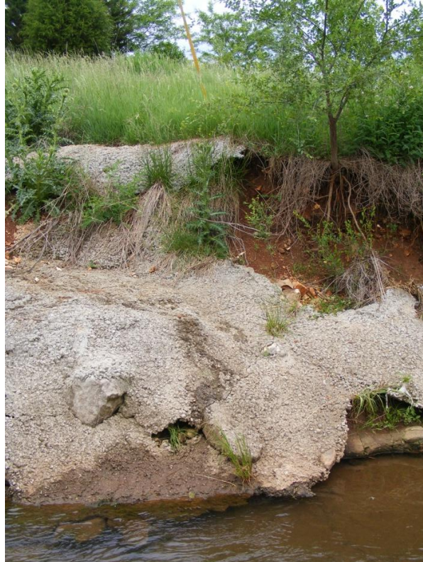
Photo 3. SR-1 cross-section #1 (station 35 ft) right bank.
