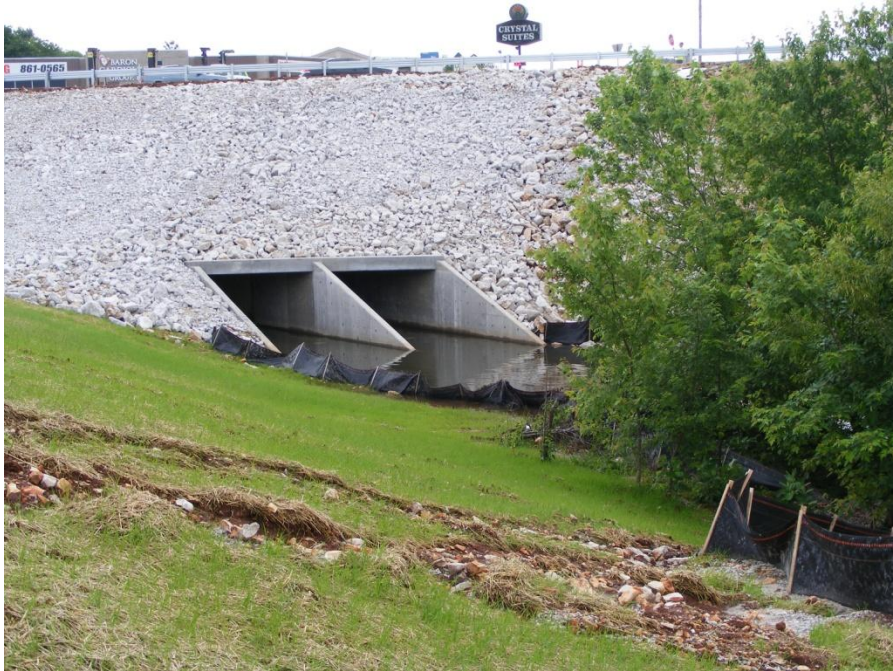
Photo 51. SR-14 downstream of National in the construction reach (station 3,050 ft).
