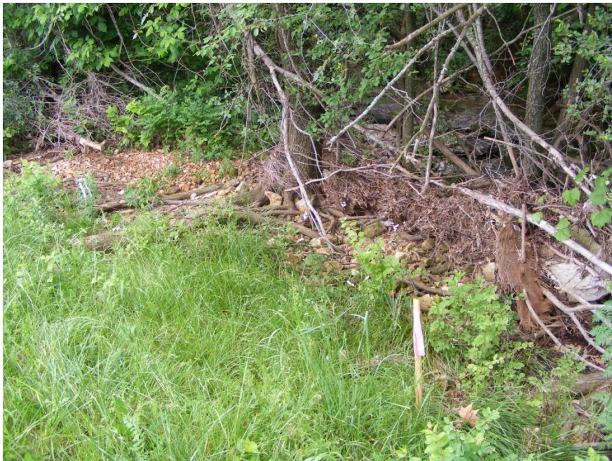
Photo 28. SR-6 gravel splay on the right bank near station 900 ft.
