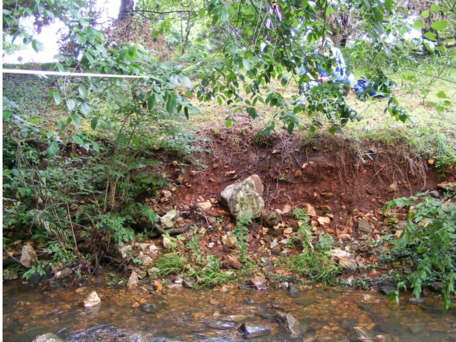
Photo 57. SR-15 section #9 (station 3,875 ft) right bank.
