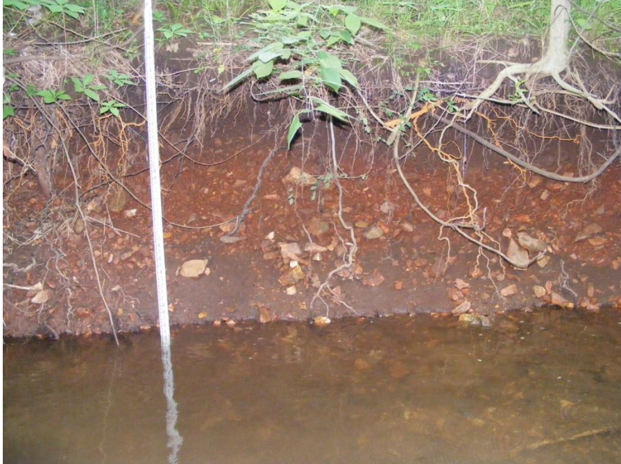
Photo 13. SR-4 cross-section #3 (station 460 ft) right bank.
