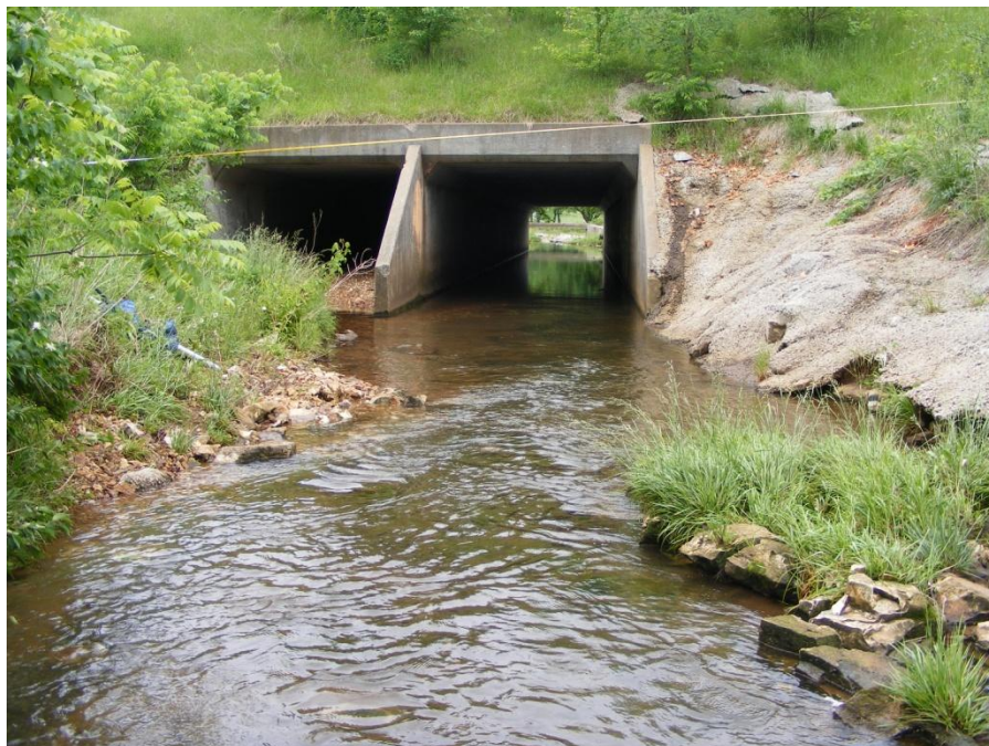
Photo 2. SR-1 cross-section #1 (station 35 ft) looking downstream at Republic Road culvert.
