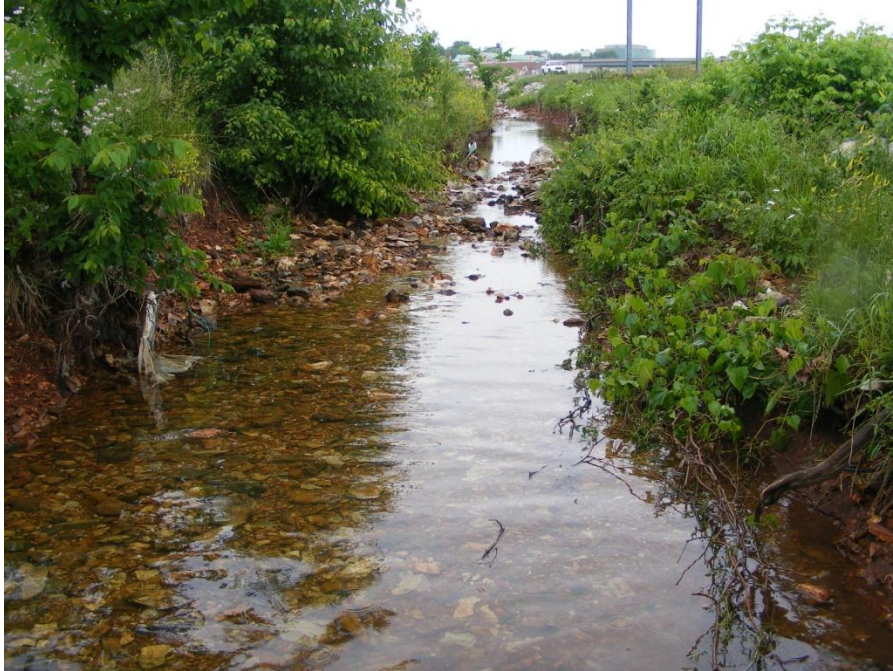
Photo 33. SR-9a looking upstream at station 1,500 ft.
