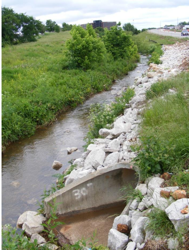
Photo 41. SR-10b looking upstream from station 1,840 ft with rip-rap along left bank falling into channel.
