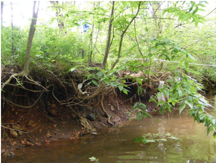
Photo 14. SR-4 cross-section #3 (station 460 ft) left bank.
