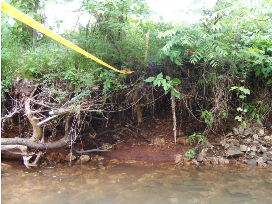
Photo 17. SR-5 cross-section #4a (station 700 ft) right bank.
