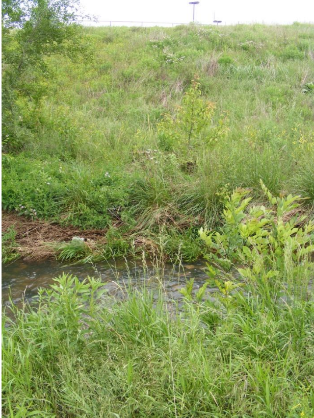
Photo 45. SR-12 cross-section #7 (station 2,210 ft) right bank.
