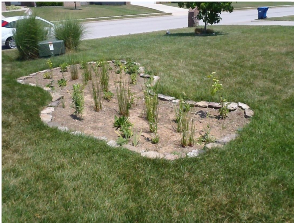
Photo 2. Example of a rain garden installed at Park Hill
