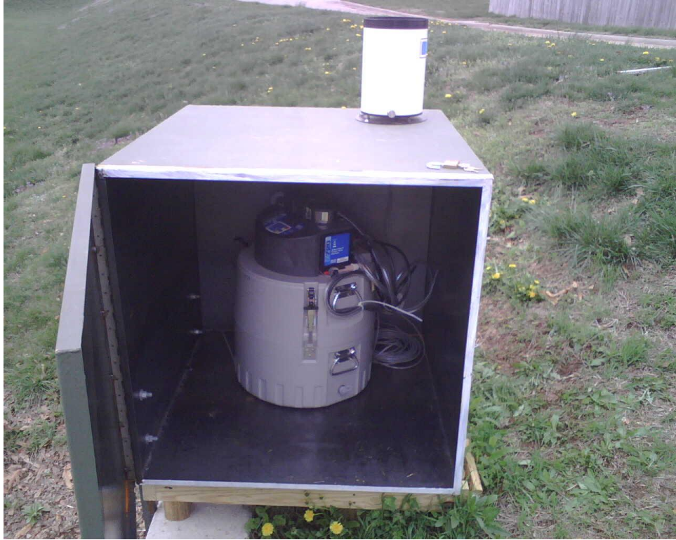
Photo 5. Installation at Park Hill Subdivision in Nixa
