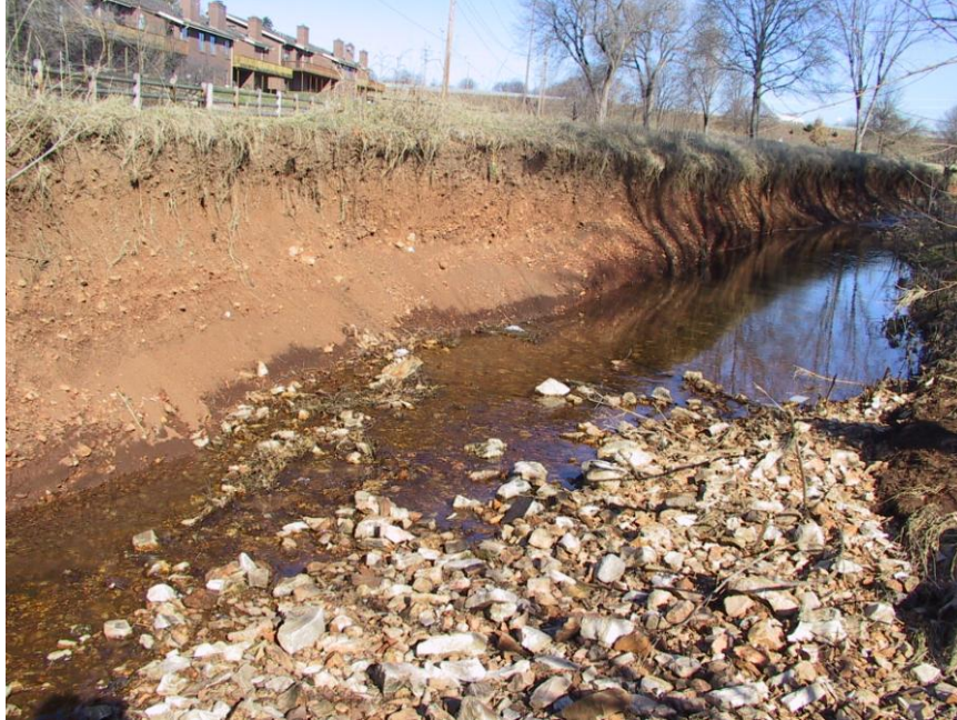
Photo 3. High bank at station 1,000 feet
