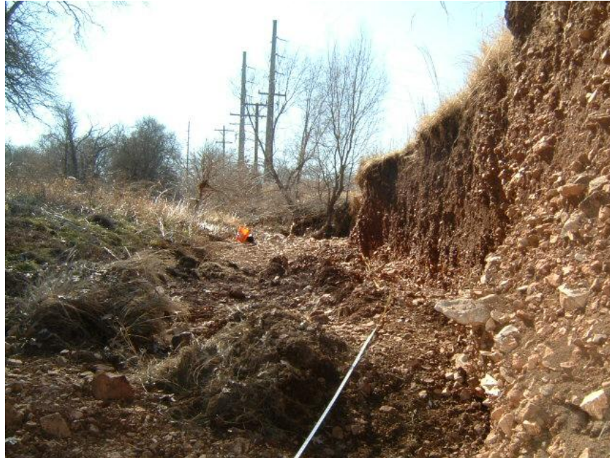
Photo 3. Bank material lying in the stream after collapse
