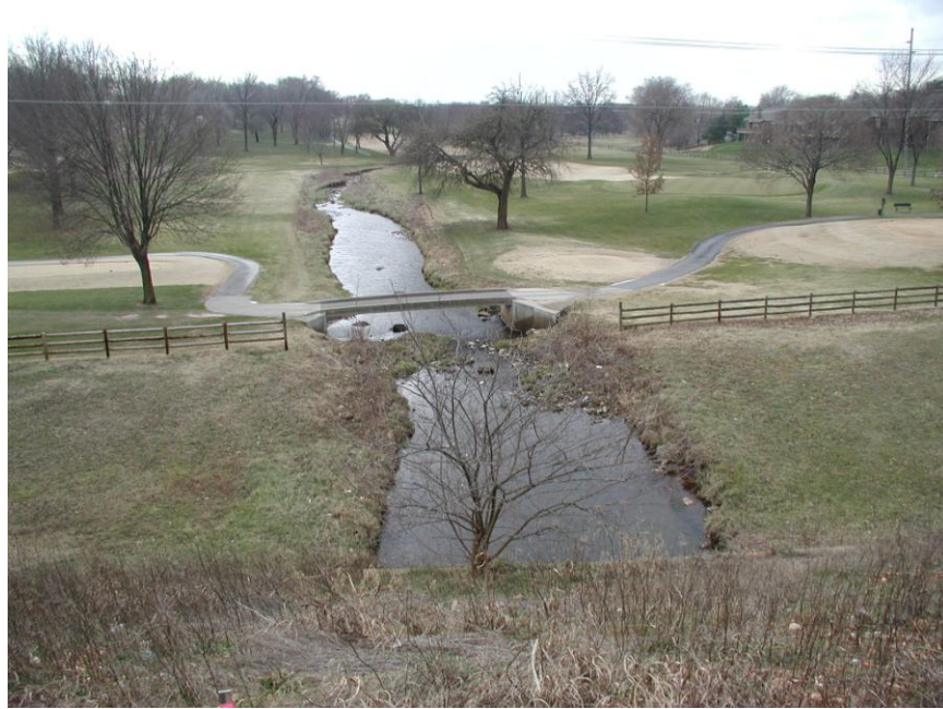
Photo 1. Looking south at Republic Road
