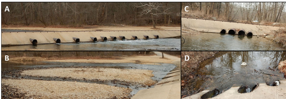
Figure 2. (A) Downstream view of the main channel crossing at Cedar Grove. (B) Upstream view of the main channel crossing showing heavy amounts of sediment deposition. (C) Downstream view of the side channel crossing at Cedar Grove. (D) Upstream view of the side channel crossing showing lighter sediment deposition. Pictures were taken February 9, 2018. Discharge at the Cedar Grove low-water crossing is 2.33 \text{ m}^3/\text{s} (Akers Ferry = 5.10 \text{ m}^3/\text{s} ).
