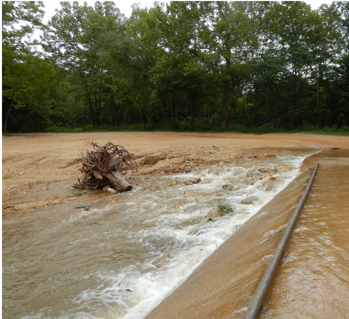
Figure 4. Image of the pseudo-fish ladder formed along the edge of the main channel crossing following heavy rainfall. The discharge at Akers Ferry is approximately 28 \text{ m}^3/\text{s} during this photo. Picture taken August 17, 2017.
