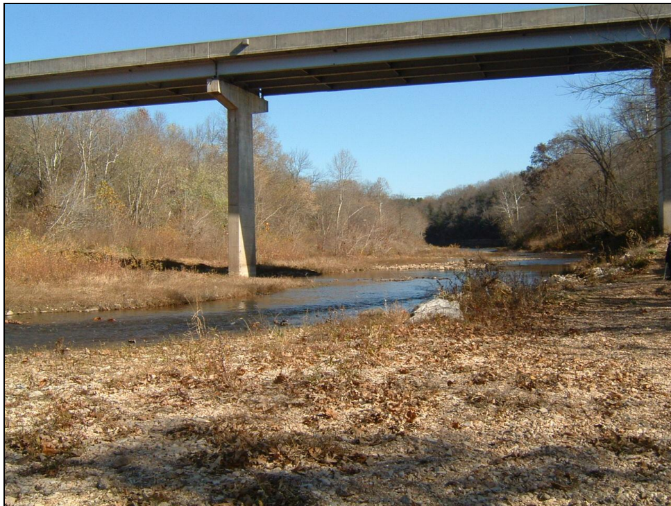
Figure 2.27: Kings River (14). Site at Highway 143 near Berryville, Arkansas (November 13, 2005)
