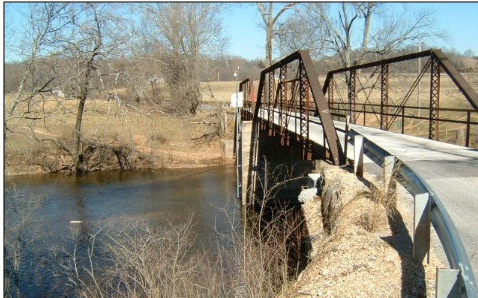
Figure 2.10: Finley Ck (5). Site at Riverdale Road Bridge (February 12, 2006)
