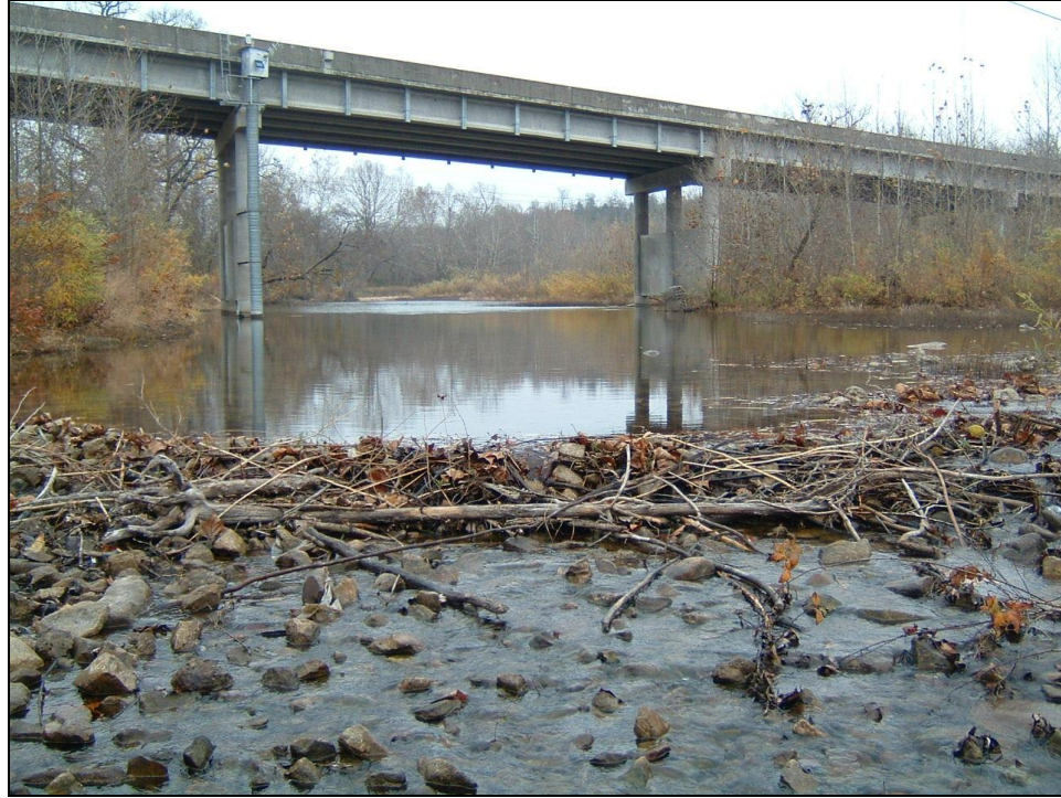
Figure 2.16: Bull Creek (8). USGS gage site with beaver dam (November 12, 2005)
