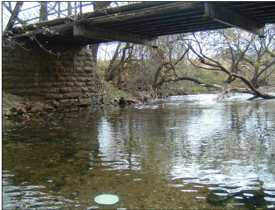
Figure 2.8: WC-at SWTP (3). Site off West Farm Road 168 (November 12, 2005)
