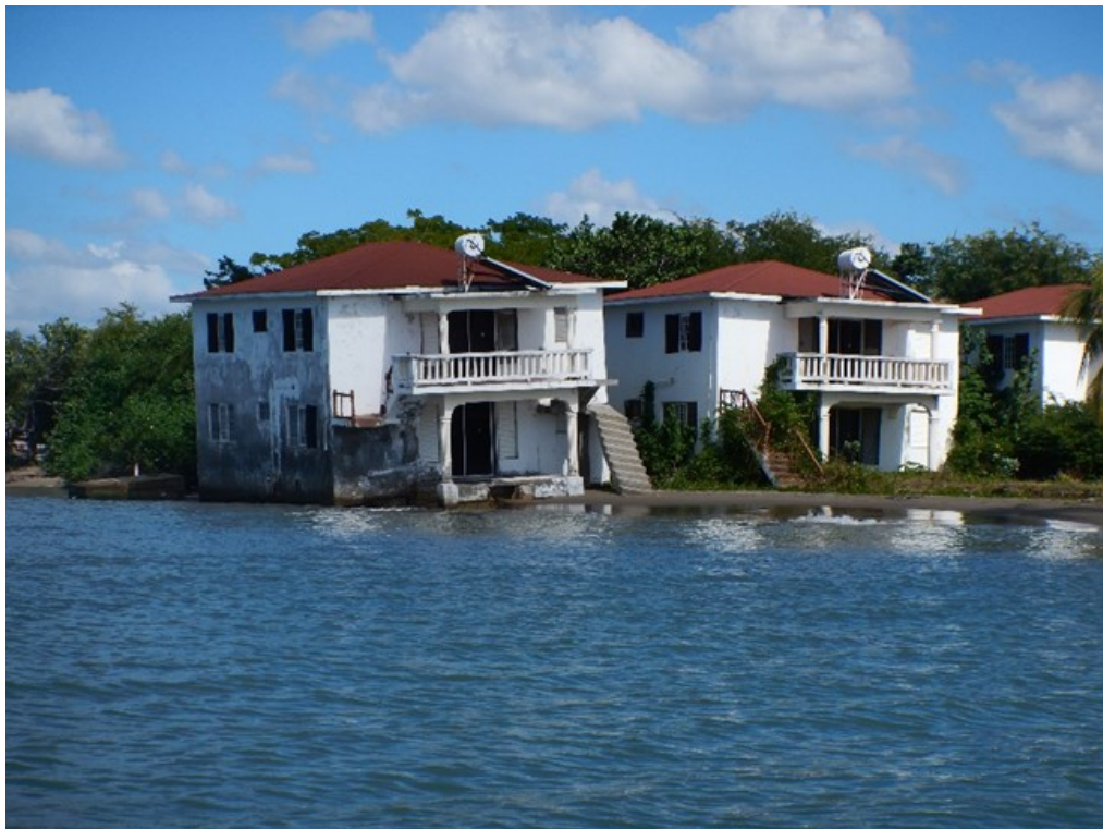
Figure 27. Property Damage Due to SLR and Shoreline Erosion. Picture taken in January, 2014.
