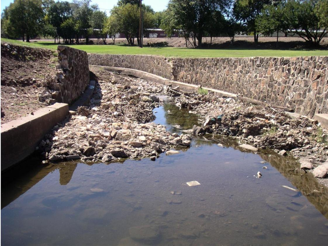
Figure 31. Failed bank armoring along Jordan Creek upstream of site 39.
