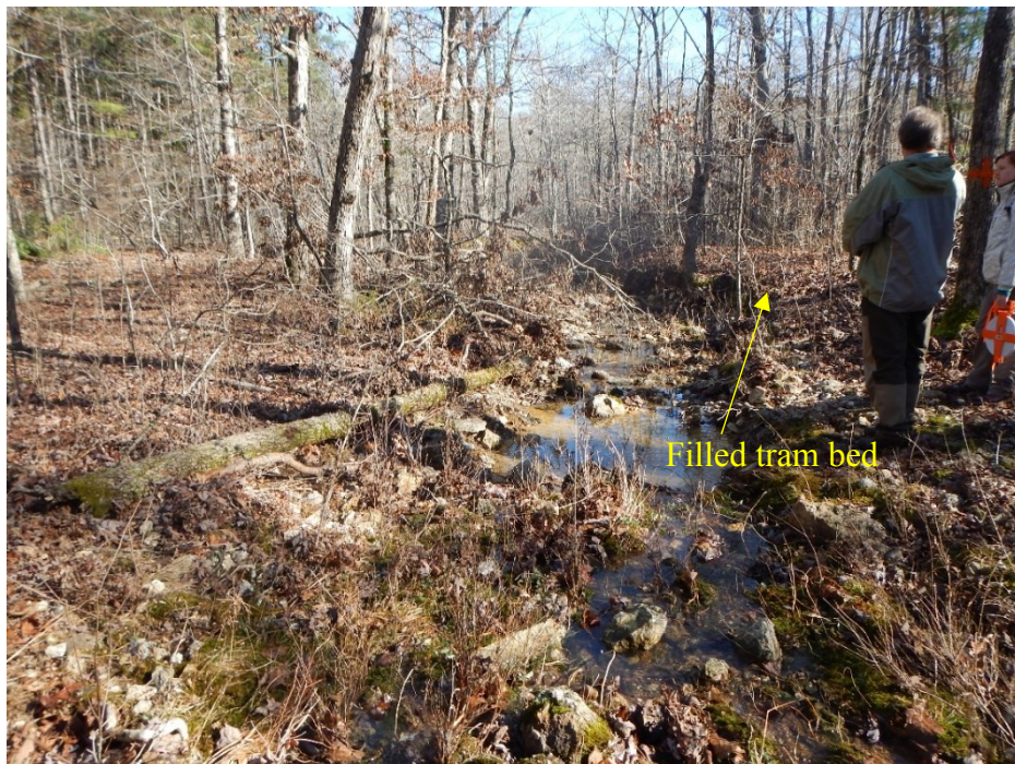
Figure 3. Filled Tram Bed Features in Tram Hollow: A.) Filled tram bed, R-km 1.17, B.) Filled tram bed, R-km 2.21. Pictures taken in December 2015 by Nick Bradley.
