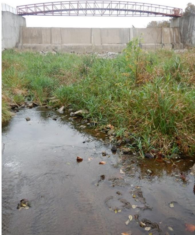
Figure 16. Valley Water Mill Reservoir seepage
