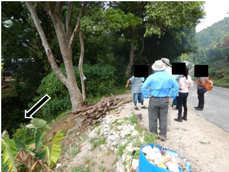
Appendix B-24. Point 21 – Gorge Right Bank/Road Fill
