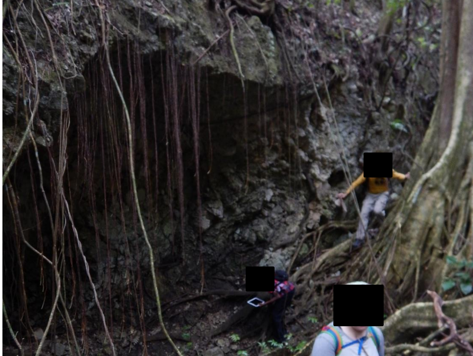
Appendix B-35. Point 30 – A “Scour Cave” on the Wall of a Bedrock Channel Along the Mid-Valley Reach Where Material Was Eroded from the Wall
