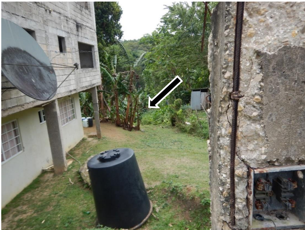
Appendix B-26. Point 22 – Upstream of Brighton Road Where the Saddle Cut in the Village of Brighton Occurred, the Depression Overfilled and Spilled over the Road
